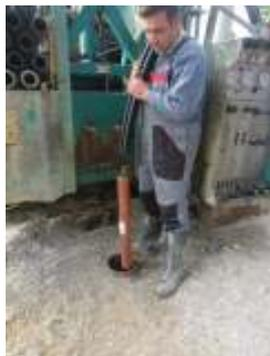
Fig. 5. Introduction of geothermal heat exchanger in the borehole.
