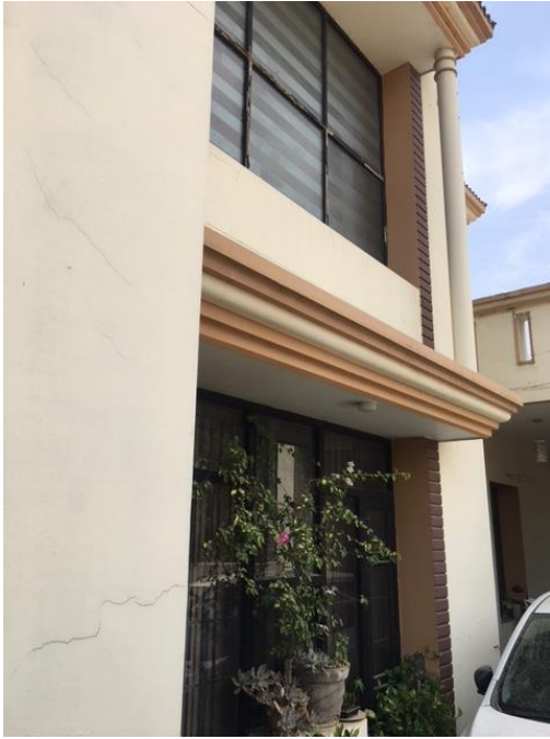
Fig.5 : Exterior openings on double height façade
