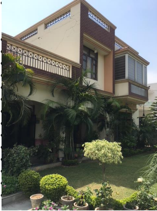
Fig.3 : Front elevation facing north-east
